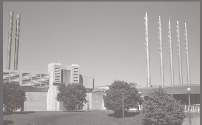
WELLINGTON HOSPITAL ENERGY CENTRE
